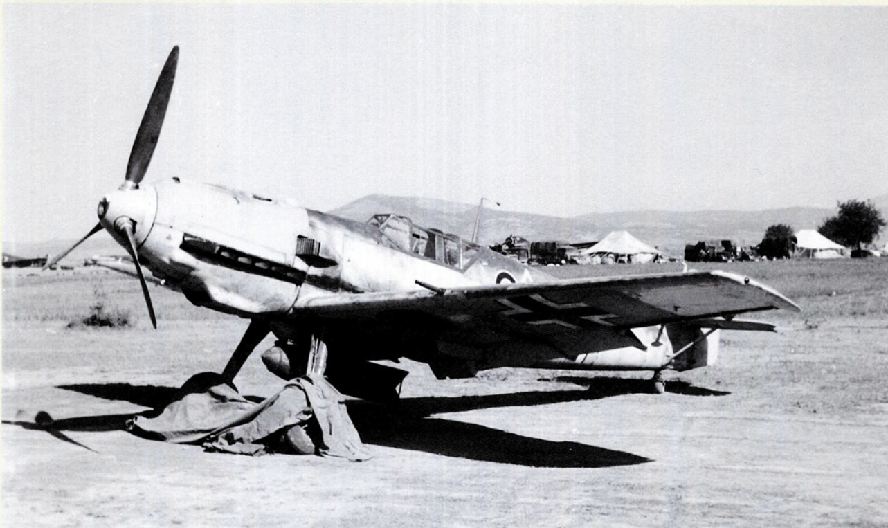
LEFT: With its tyres protected from the sun, this Bf 109 E of 5./JG 77 at Molaoi in May 1941 has already been loaded with a 250 kg bomb prior to a sortie to Crete. The spinner, nose, rudder and wingtips have been painted yellow, but the yellow on the leading edge of the wingtips is badly eroded as a result of the abrasive dust on Balkan airfields.
